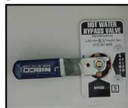
**Figure 11-10. Water Heater Bypass**
