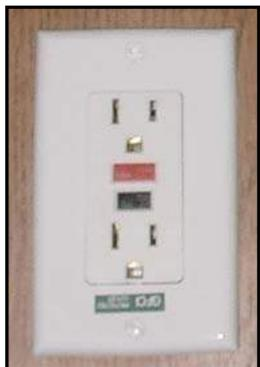
**Figure 7-14. Ground-Fault Circuit Interrupter (GFCI)**
