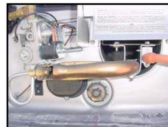
**Figure 4-16. Water Heater Drain**
