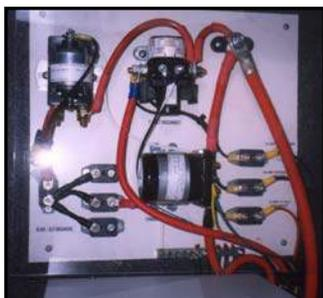
**Figure 7-19. Resettable Circuit Breakers**
