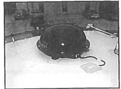
Figure 4-19. CB Antenna Installation
