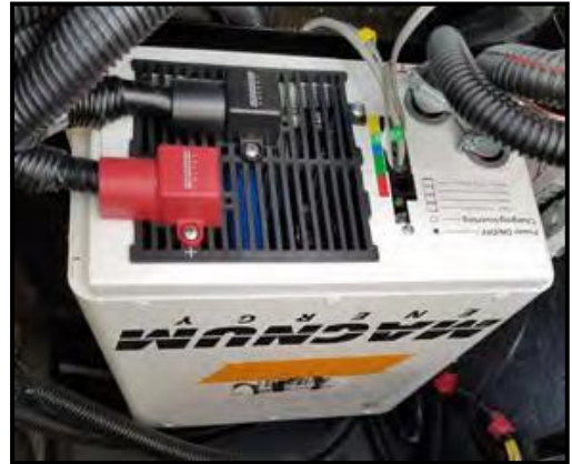
Figure 9-15: Converter/Inverter
