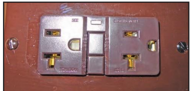
Figure 9-12: GFCI Receptacle
