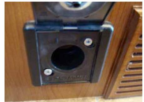
Figure 13-12. Vacuum Hose Coupling
