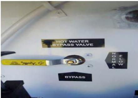
Figure 11-9. Water Heater Bypass System
