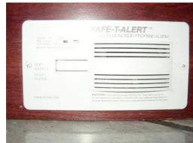
Figure 3-6. CO/LP Gas Detector
