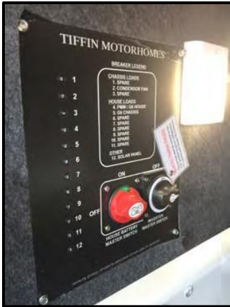
Figure 9-13: House Battery Disconnect Panel
