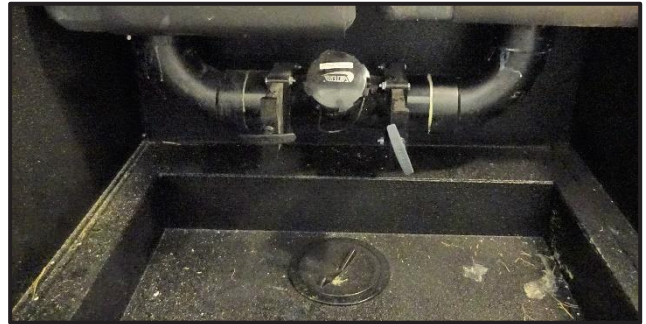
Figure 13-12: Sanitation Coupling
