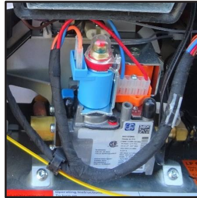
Figure 5-8: Water Heater Relief Valve
