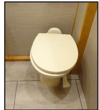
Figure 13-10: Toilet Pedal Flush Lever
