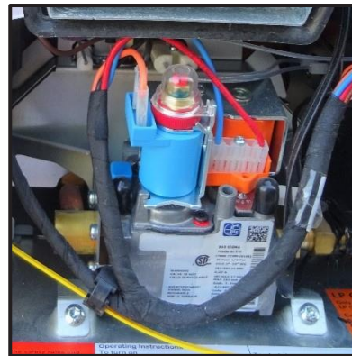
Figure 5-8: Water Heater Relief Valve
