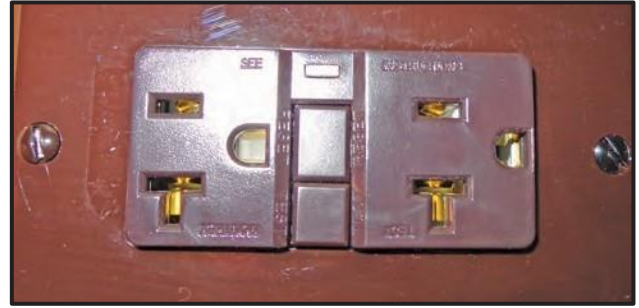
Figure 9-5: GFCI Receptacle
