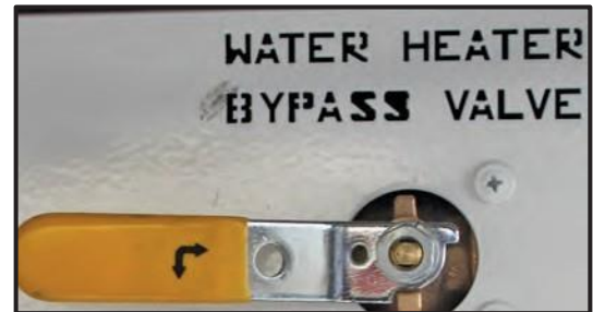
Figure 13-9: Water Heater Bypass System
